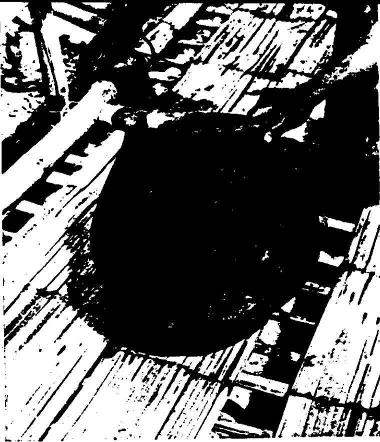
Detail of construction of Hanunoo bamboo house. The floor is of bamboo poles beaten flat. Cooking pot was made by the neighboring Buid. Their pottery is a major item of trade with the Hanunoo, who, in turn, supply the Buid with salt and other items from the coastal region.
